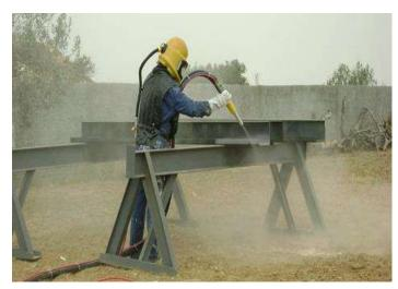
It consists of scouring the surface by projecting an abrasive through a nozzle at high velocity and under high pressure leading to:
